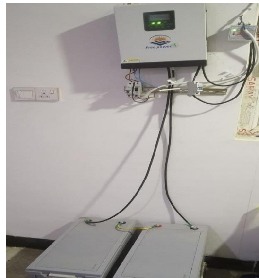
Figure 2: Full Solar system showing the inverter device and the batteries
