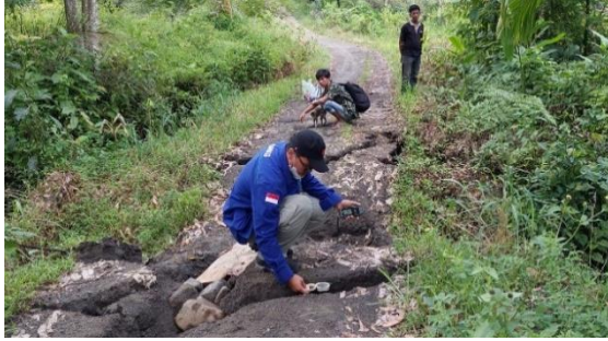
Fig.6. Ground failure at the hills of Mt.Talamau (Kajai Village)
