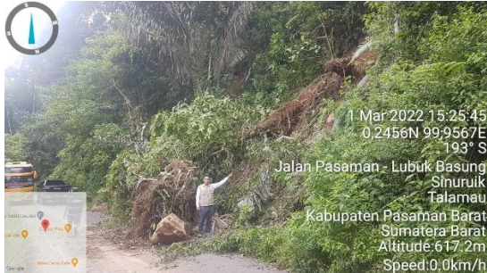
Fig.8. Soil Landslides at Talu Village
