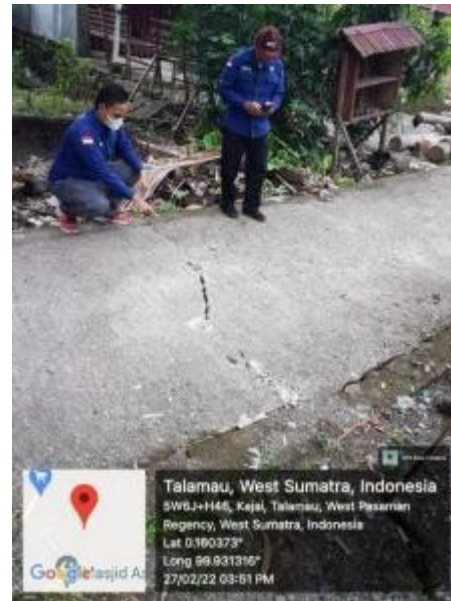
Fig.12. Ground failure at residential area Kajai Village
