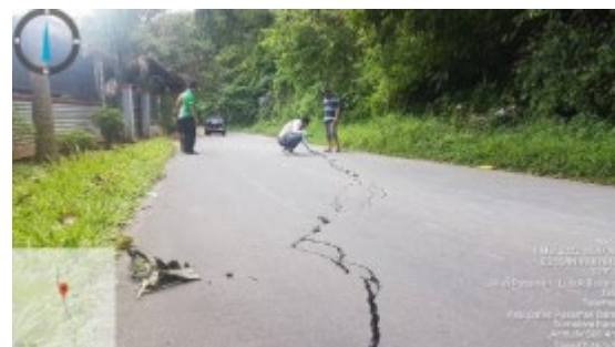
Fig.9. Ground Cracking at Talu Village
