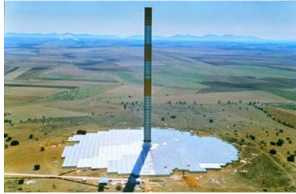
Fig .(1) Solar Chimney In Manzanares In Spain[7]
