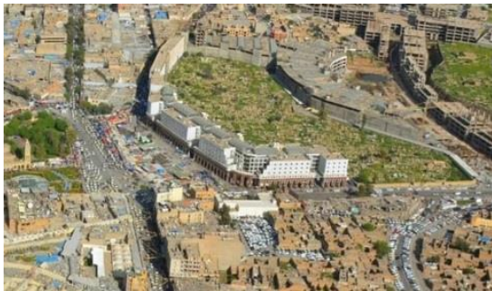
Figure.3: Shows Neshtiman Complex in Erbil City center
